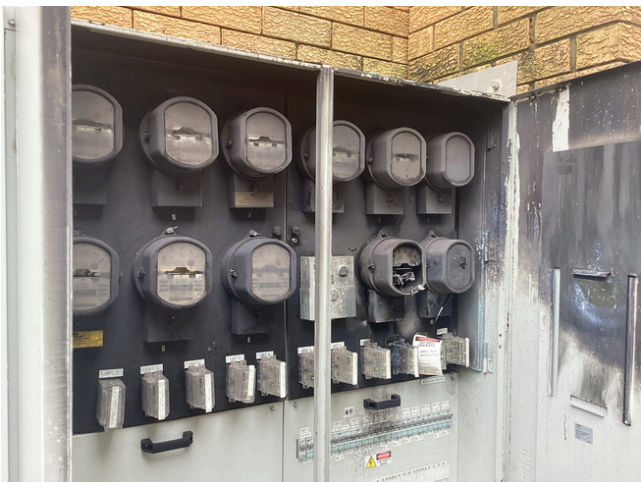
Switchboard after a fire. Source: Ocean Realty
